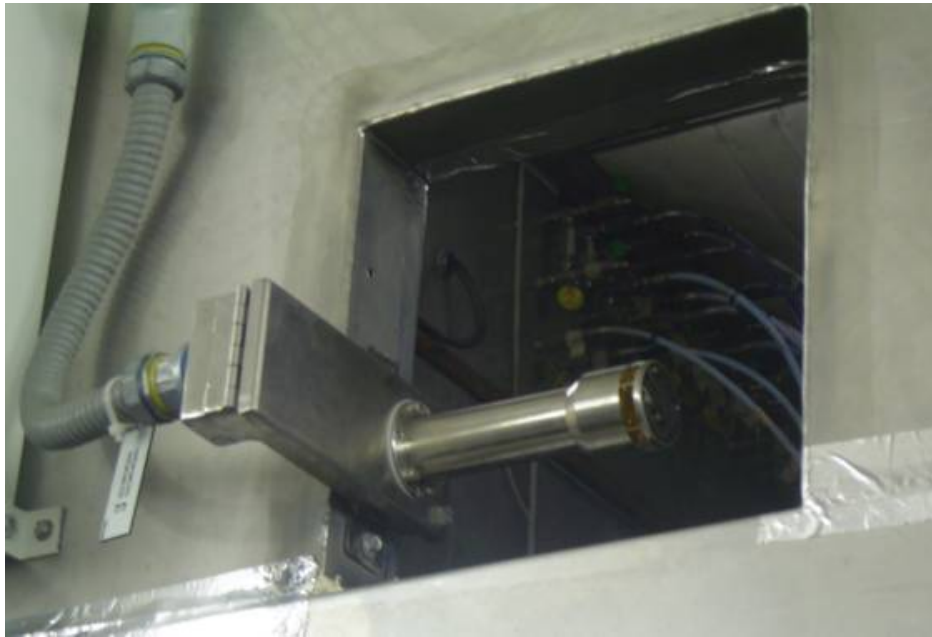
Proprietary, high-accuracy Ultrasonic airflow sensor installed in a paint booth
