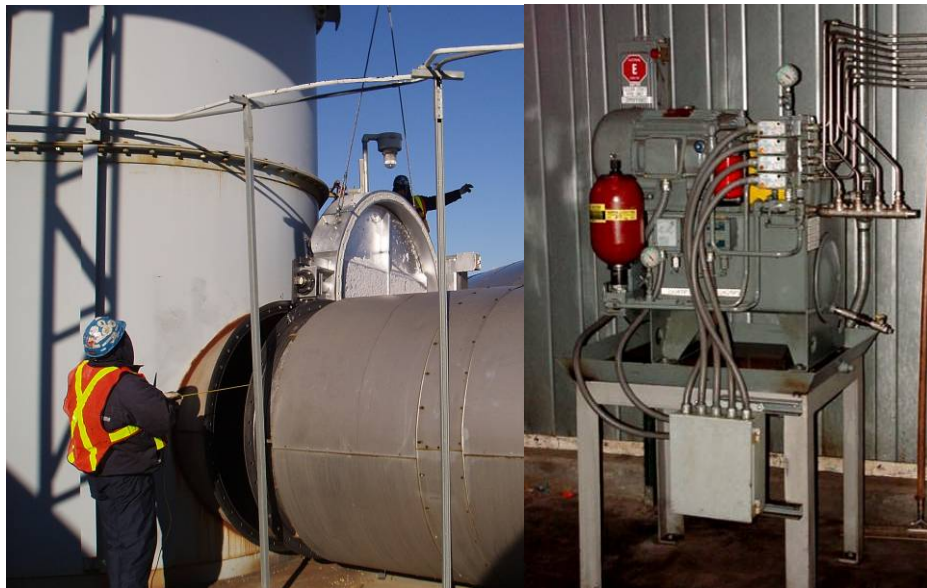
Upgrades to Mechanical Dampers and Hydraulic Actuation System
