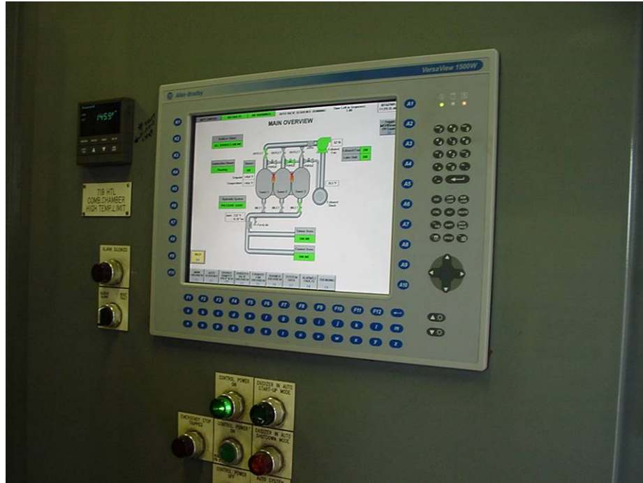
New PLC control system with a Human Machine Interface (HMI)
